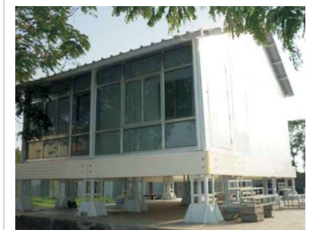
Prefabs with knocked down flooring
