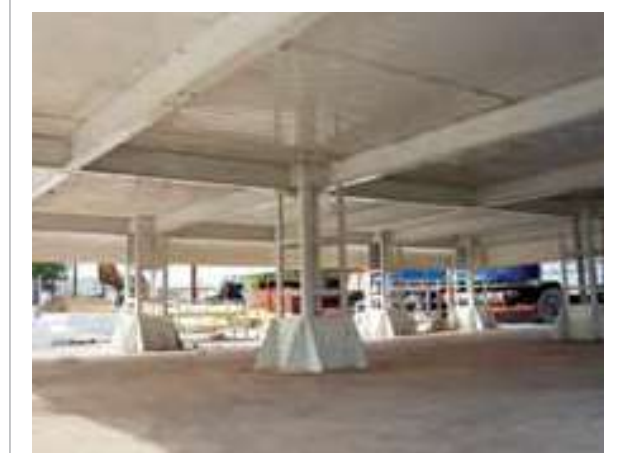
Prefabs with knocked down flooring
