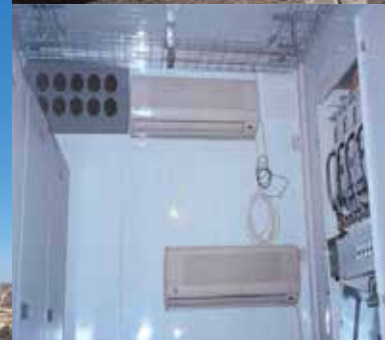
Electrical mounting and equipment using aluminium alloy C-rails
