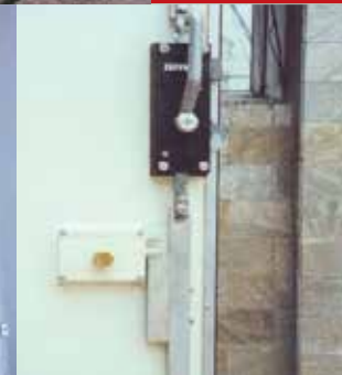
Zep door with a three way espagnolette locking system
